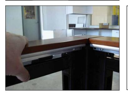
Be sure topcaps are flush with top tile retainers. Note, Radius Retainers and Linear Retainers function the same way.
